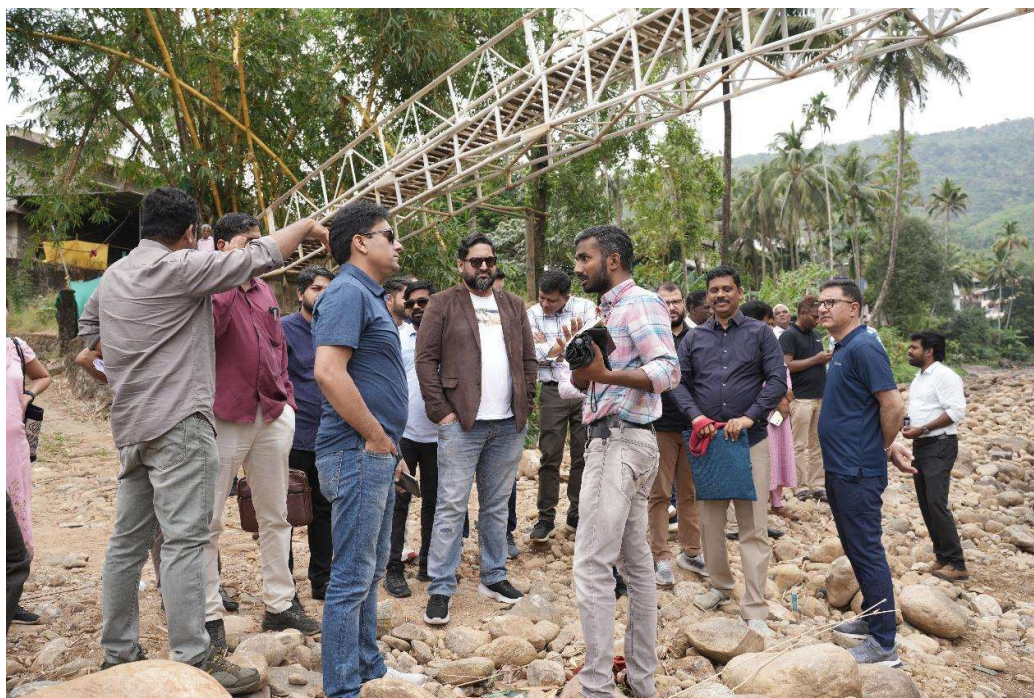
Visit to Landslide Sites as Part of the Customised Regional Training Programme on "Disaster Risk Mitigation & Management" held at Ernakulam, Kerala, for IAS Officers and Senior State Civil Service Officers, organized by KSDMA from 29th January to 1st February 2025.
